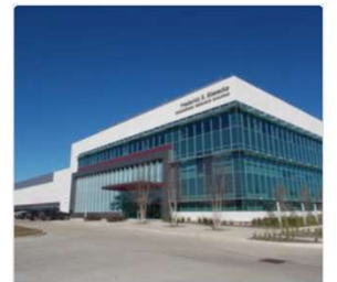
Western Smart Manufacturing Innovation Center
